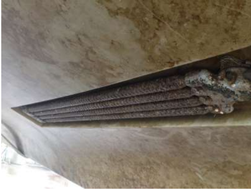
4 The keel cooler prior to removal and cleaning.
